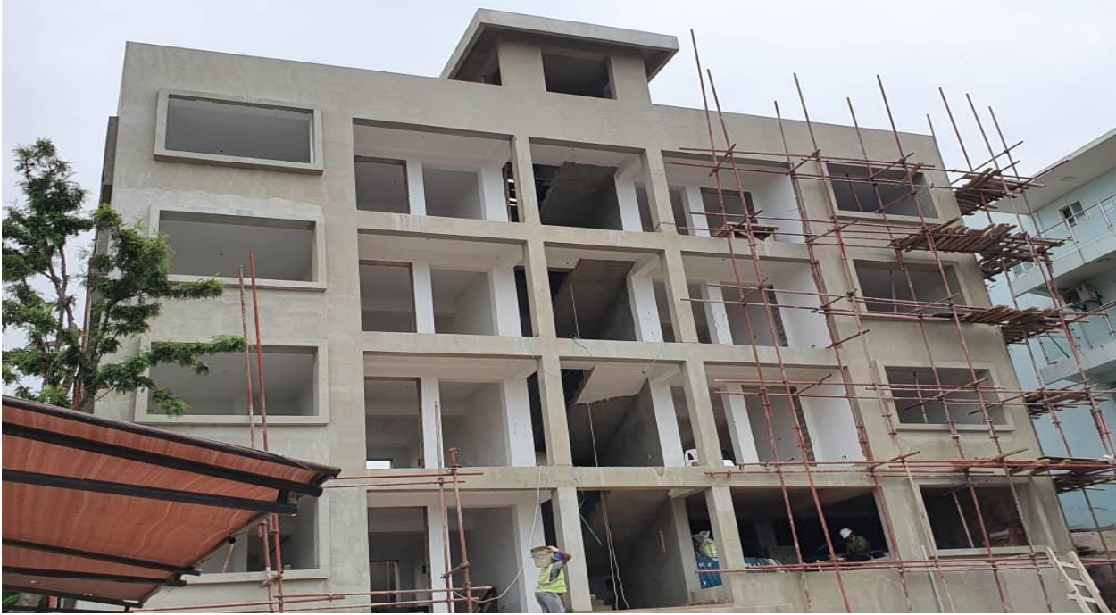
Office building on progress
