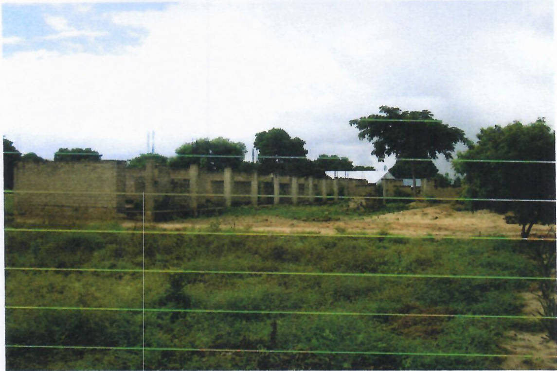
School Building 2 (Semi- developed)
