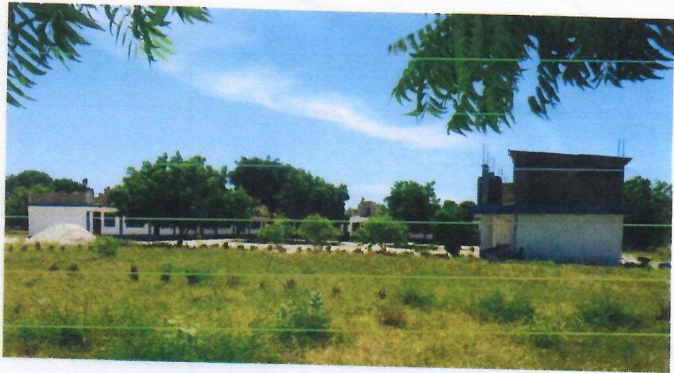
School Building 2 (Semi- Developed)
