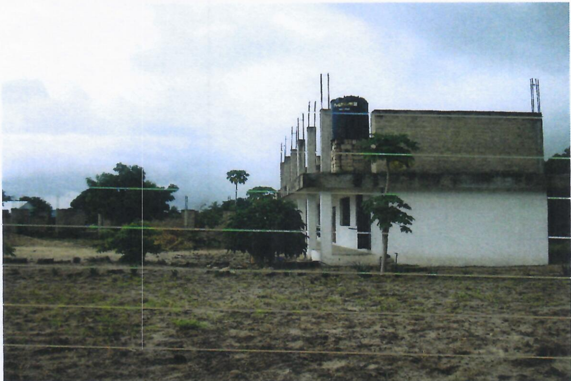
Section built up to First Floor
