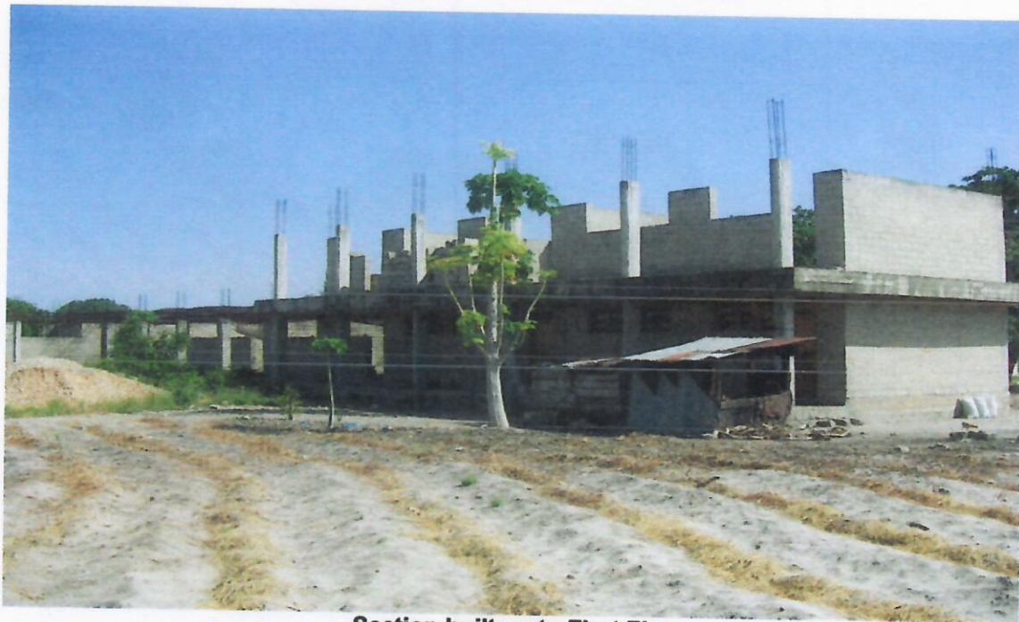
Section built up to First Floor
