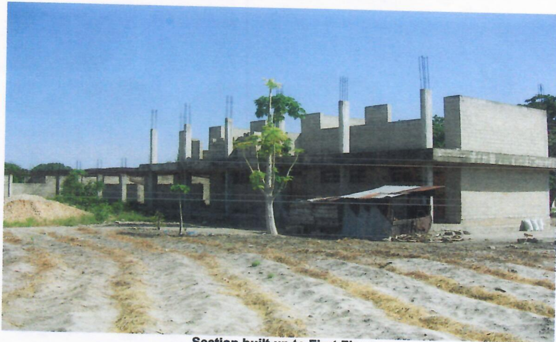
Section built up to First Floor
