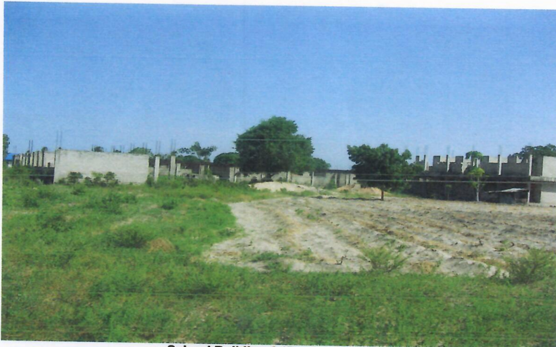
School Building 2 (Semi – developed)
