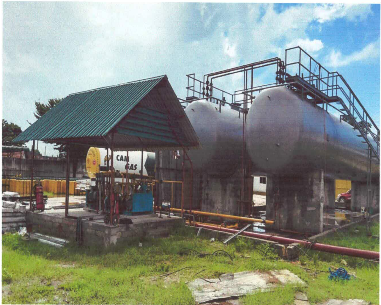
Figure 1. Construction on progress – Cam Gas Kurasini LPG Mini filling Plant
