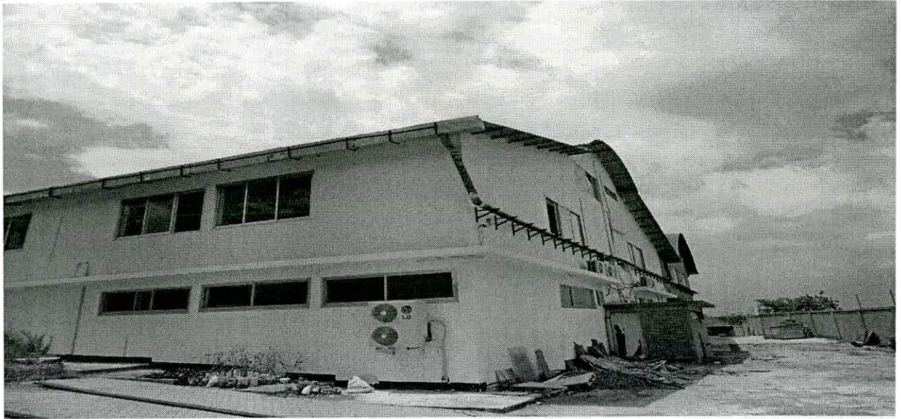
Yuko's Main Building
