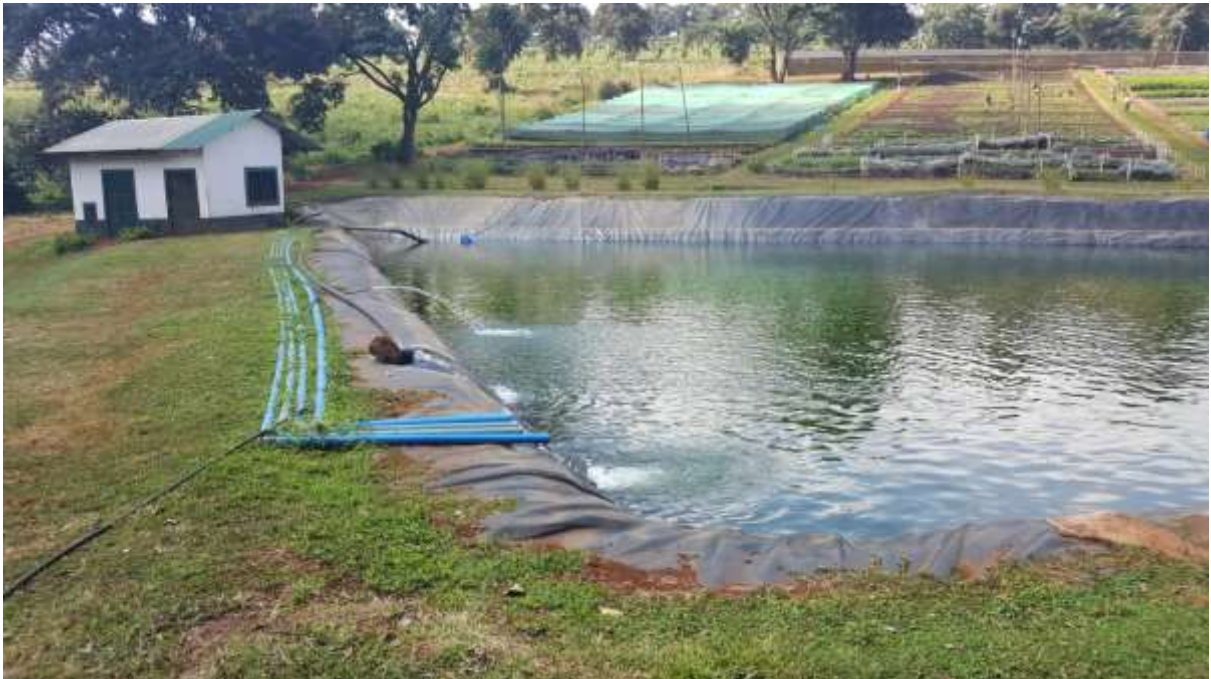
Water Storage Reservoir & Pump House
