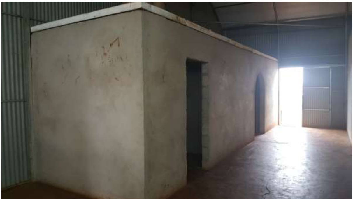
Ablutions (Under construction)
