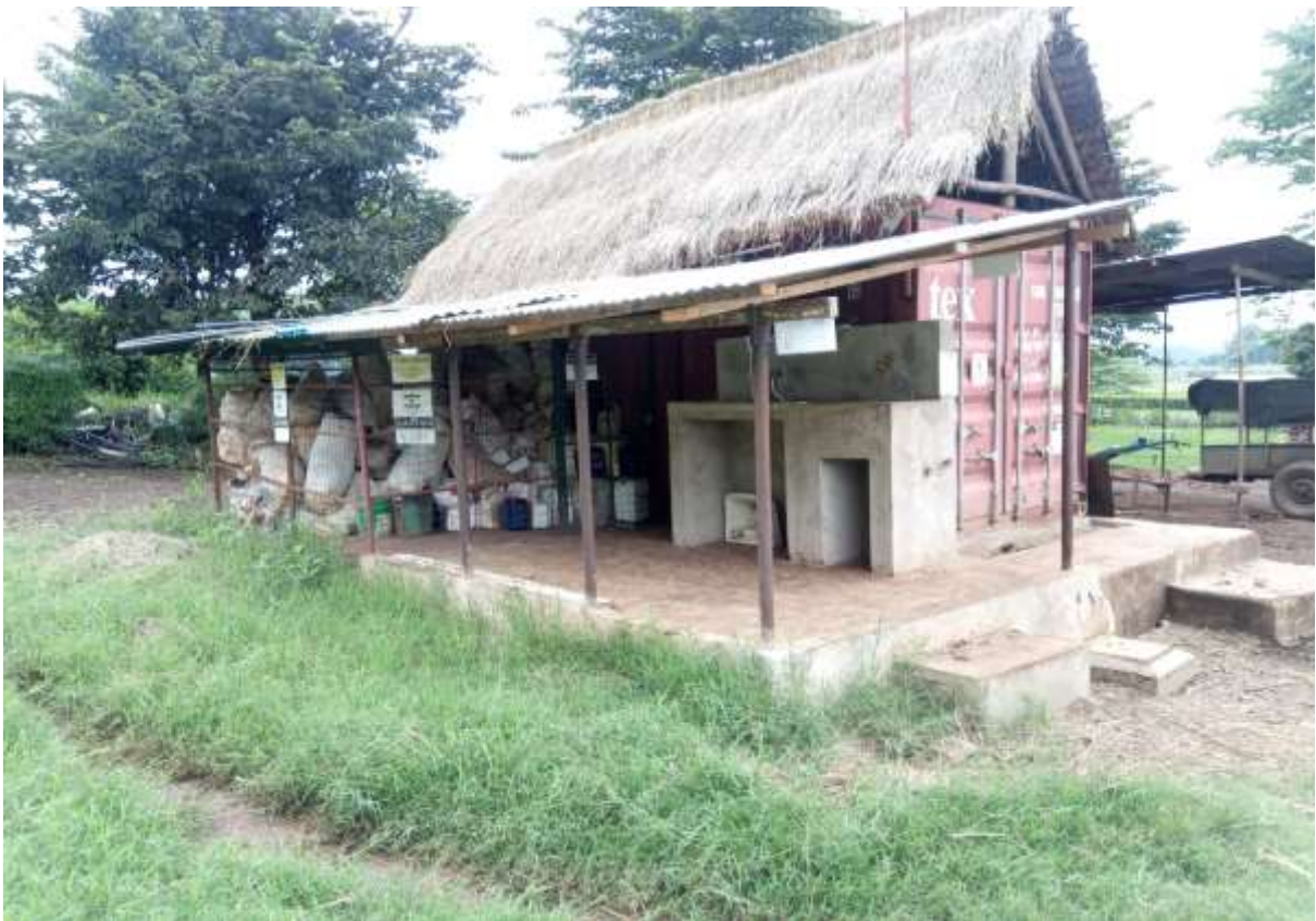
Chemical Mixing Area
