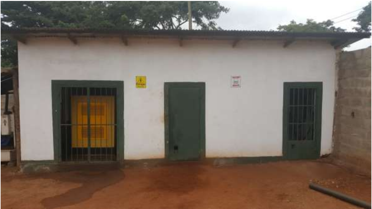
Power Supply Building.
