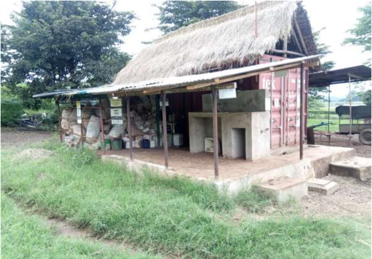
Chemical Mixing Area
