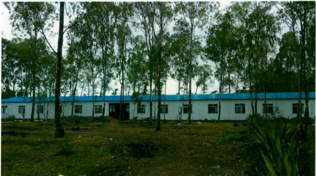
One of the complete building during the construction phase one.
