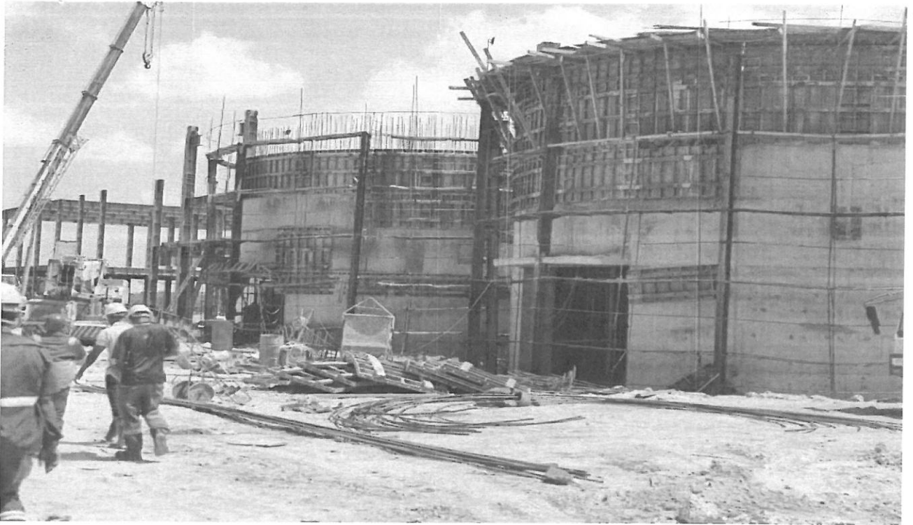
On-going construction of the cement grinding factory at Maweni, Tanga City
