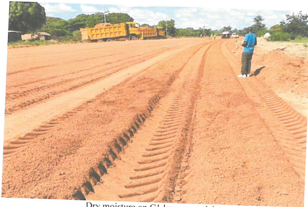
Dry moisture on C1 layer material
