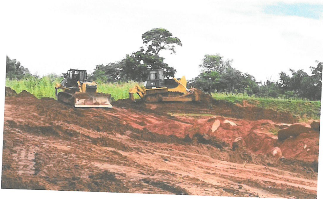
Borrow Pit Trimming at Km36
