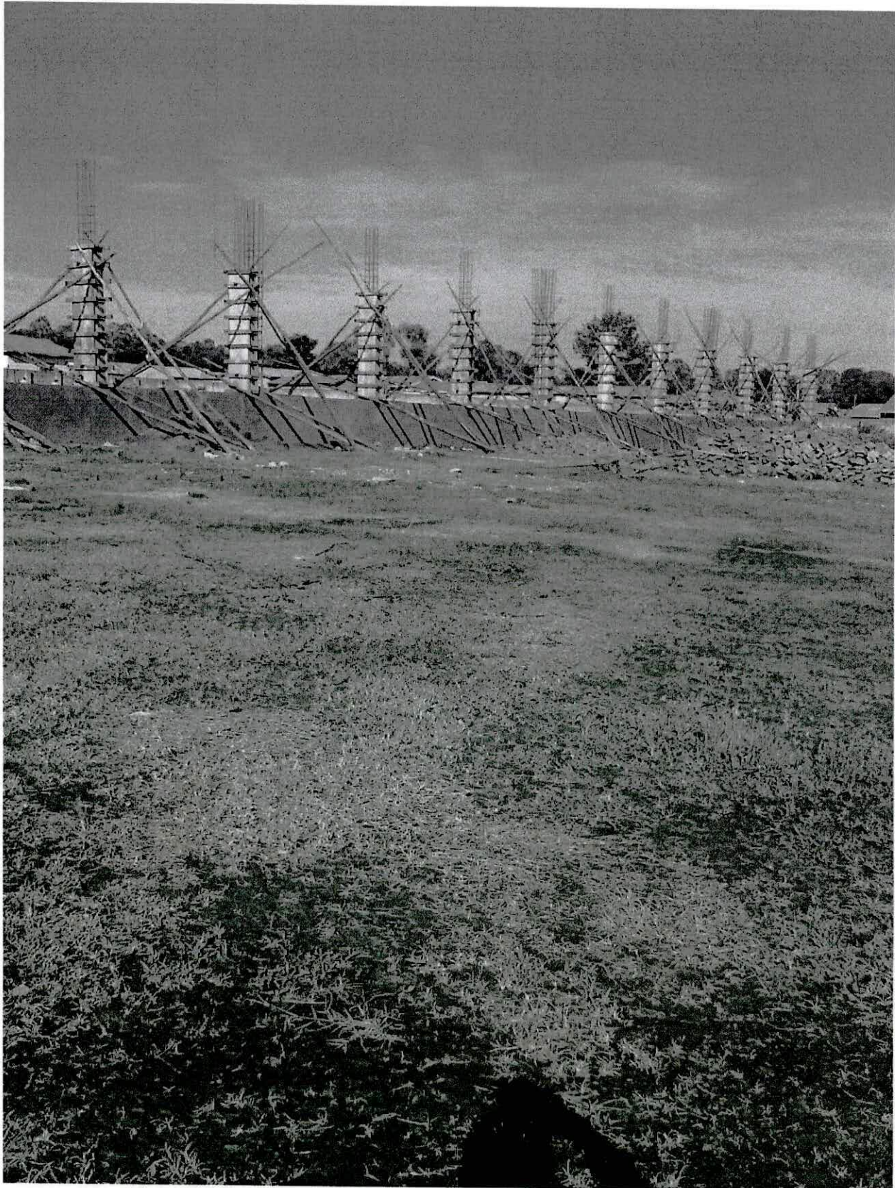
View of Warehouse/Godown Buildings under construction
