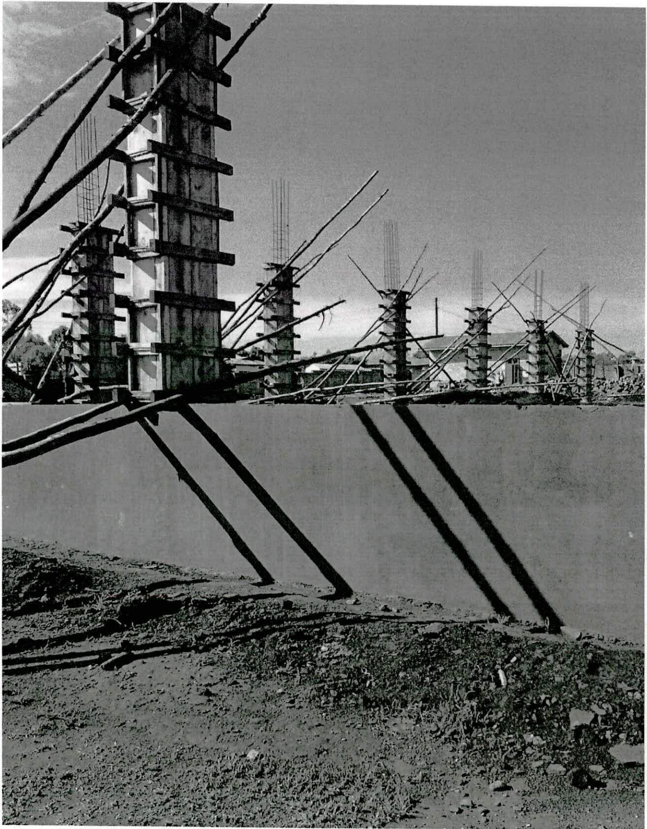
View of Factory Buildings under construction
