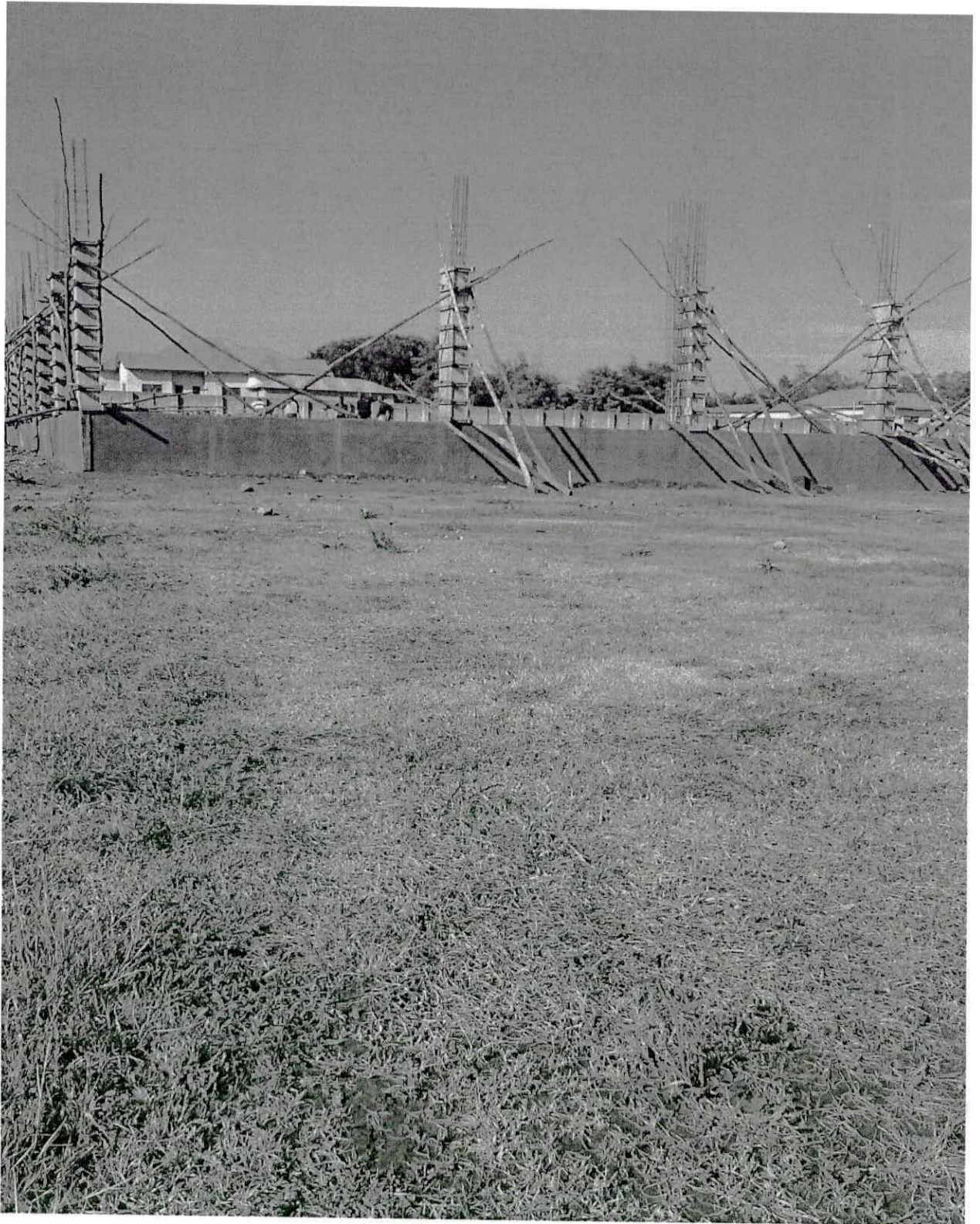
Warehousing/Storage Section under construction
