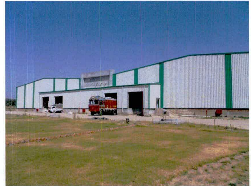
Out side view of Plant
