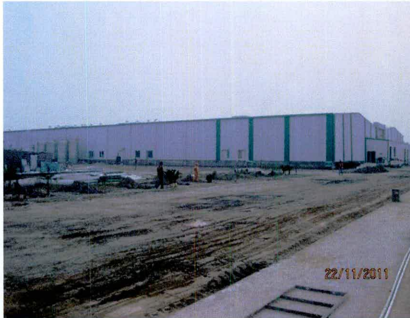
Side view of Plant
