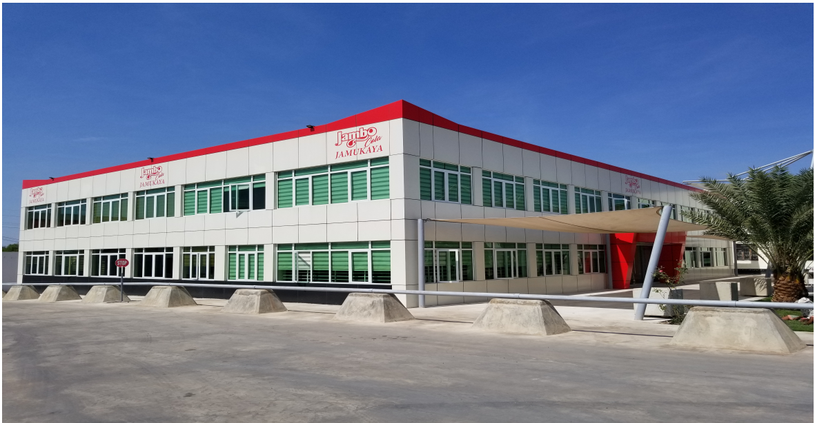
A well established office with fully set of feniture and fittings
