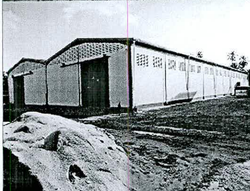
Front Elevation of an Industrial Building
