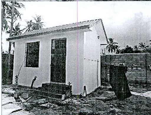
Front & Side of the Elevations of the Generator House
