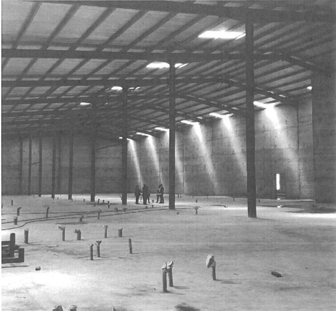
Photo 3: Installation of Production lines
