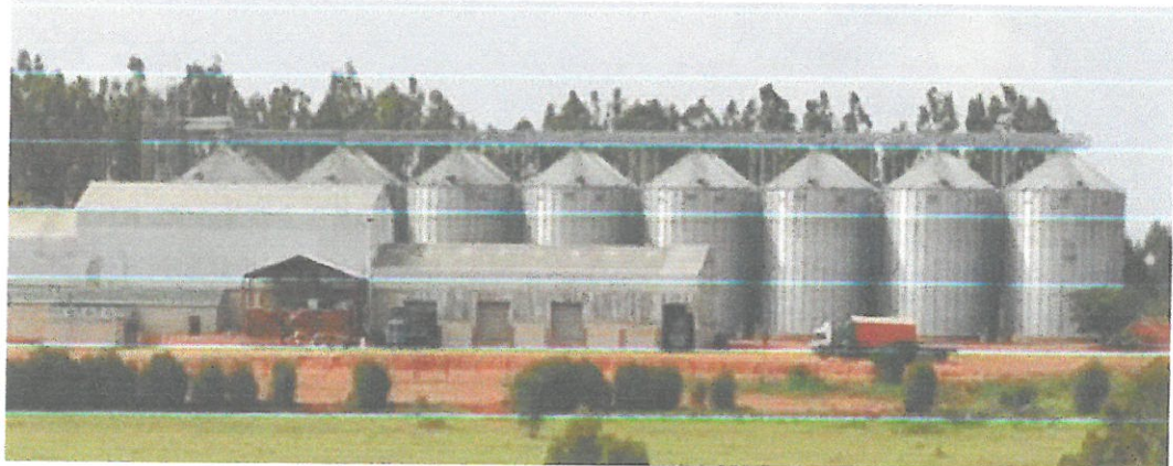
Silos and Feed Mill Complex
