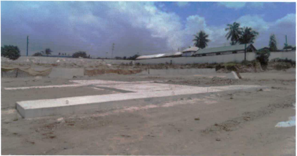
FOUNDATION FOR MOBILE BATCH PLANT ELKON MIX 60 BEAR
