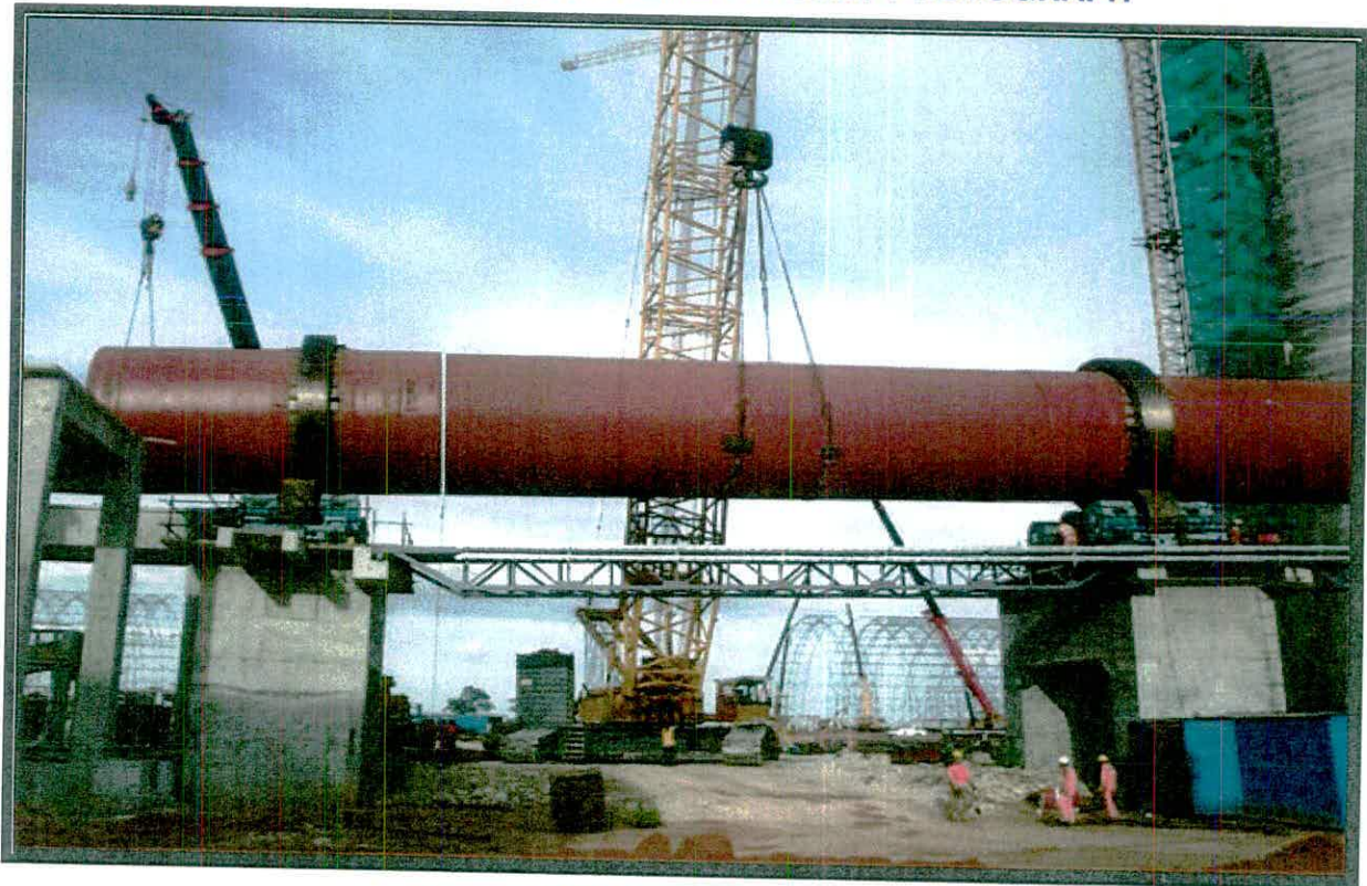
ROTARY KILN UNDER ERECTION
