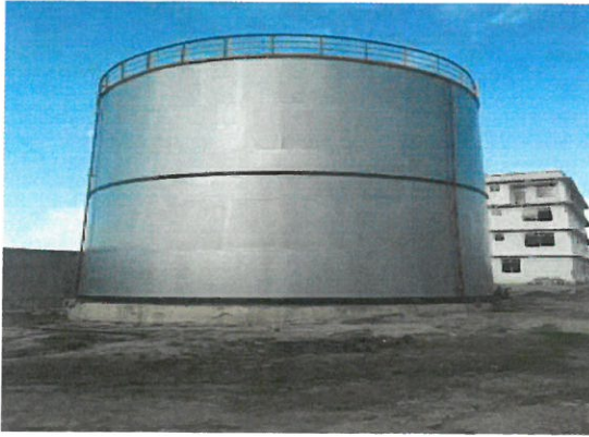
c) Water storage tank with office block in the background.
