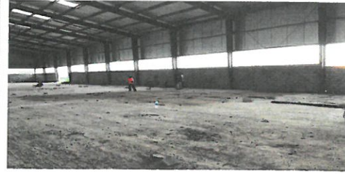
b) Factory building : Interior Setting out for drainage pipeline
