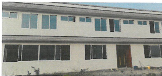
e) Technical Staff Hostel : Aluminum windows fitting Completed
