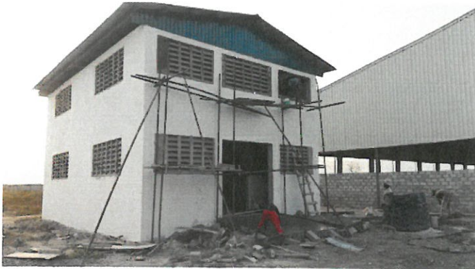
d) Boiler room under construction
