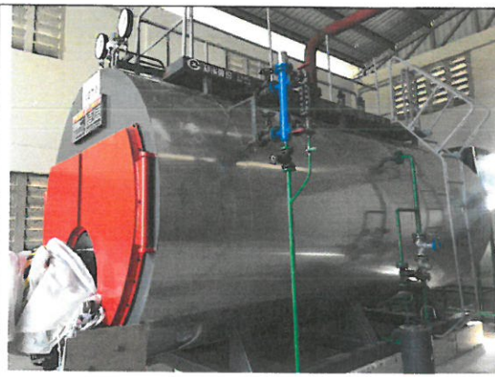
Figure 2 installation of 8tons boiler
