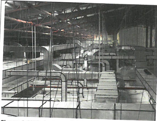
Figure 4 AHU ducts works on progress
