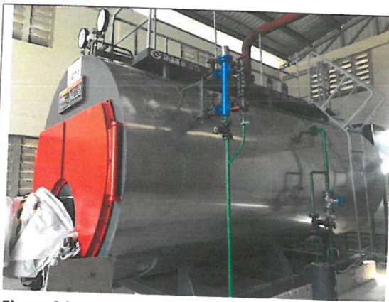
Figure 2 installation of 8tons boiler
