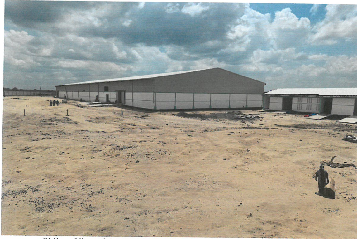
Oblique View of the Factory Building and Powerhouse; January 2021
