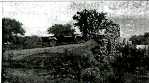
Construction of the Feeding Ramp is 75% Complete.
