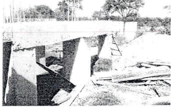
Construction of Crusher Bed as was in Progress
