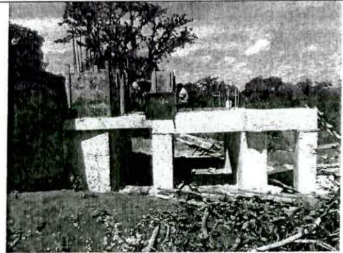
Final Touches for Finalization of Crushing Bed as was in Progress
