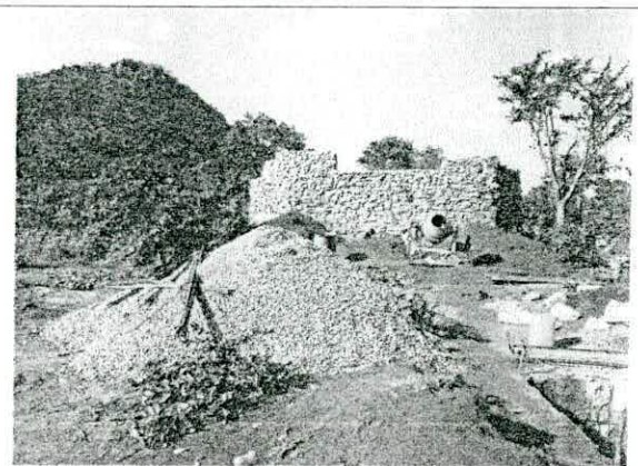
Preparatory Works for Construction of the Foundation
