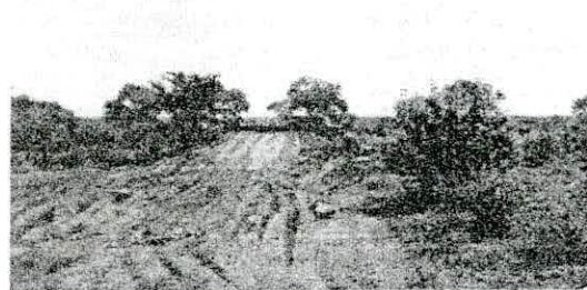
Front View of the Feeding Ramp under Construction
