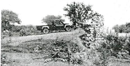
Construction of the Feeding Ramp is 75% Complete.
