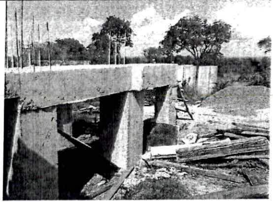
Construction of Crusher Bed as was in Progress
