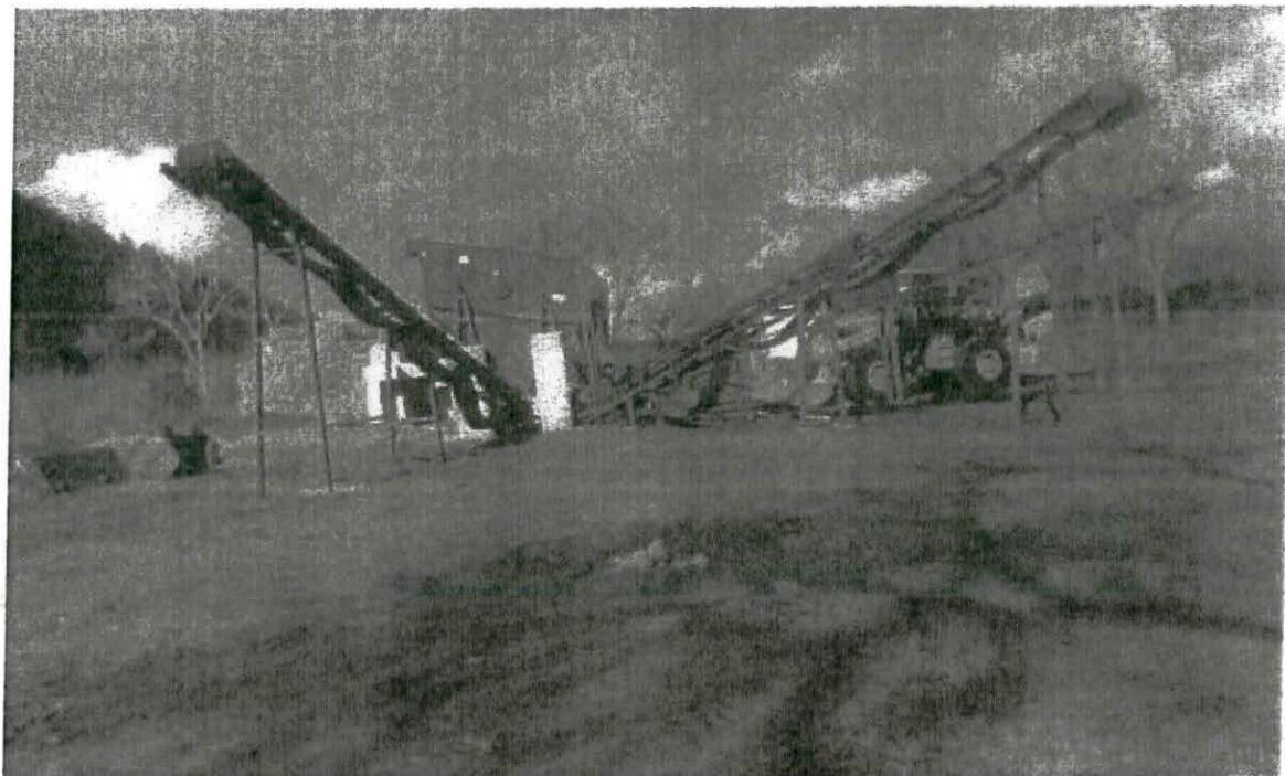
LAYOUT OF THE CRUSHER AT ALMOST 90% COMPLETION
