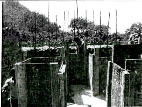
Form working to the Feeder/Crusher Bed as was in Progress
