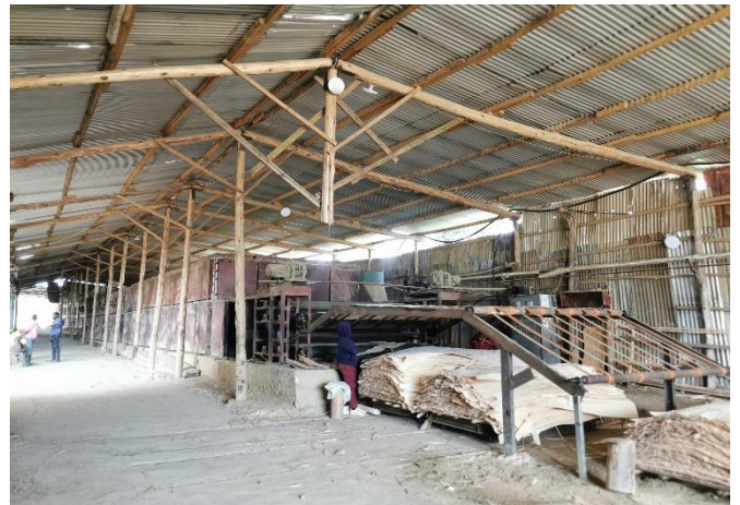
Pic 4. Drying Machine Area
