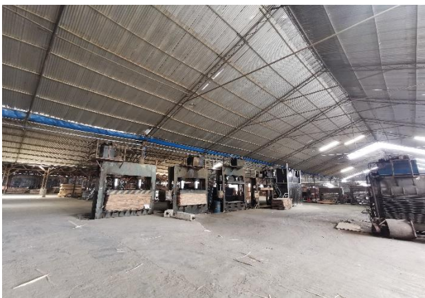
Pic 5. Marine & Plywood Workshop1
