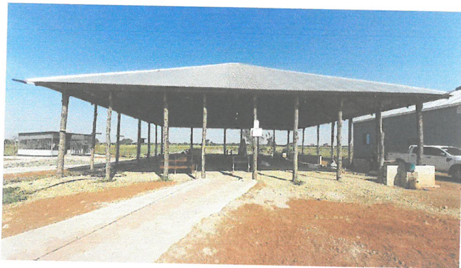
Shaft shed cover
