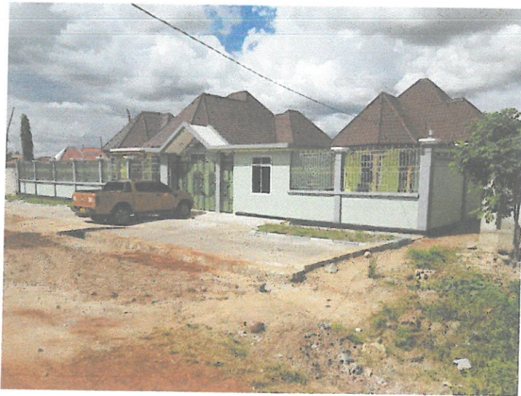
Office and residence Kahama City
