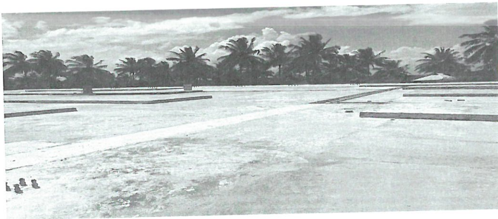
(Concrete base as found at the site)
