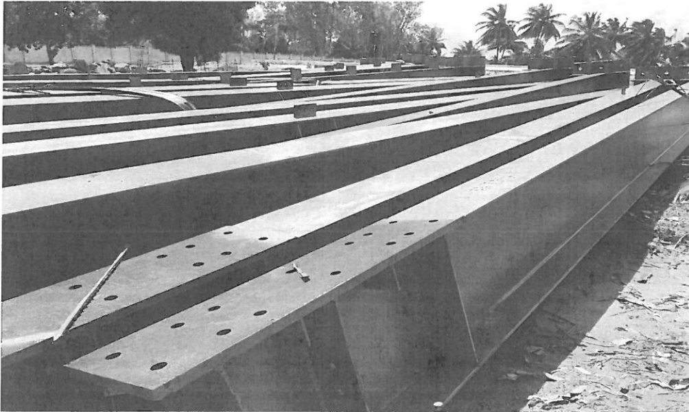
(steel structural beams imported for factory construction found at the site)
