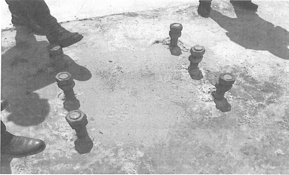
(view of the constructed concrete base)
