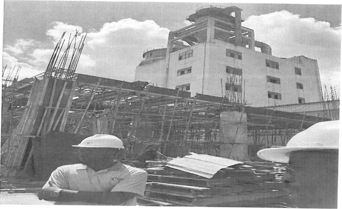
Additional 20,000 tons capacity washing powder project in progress
