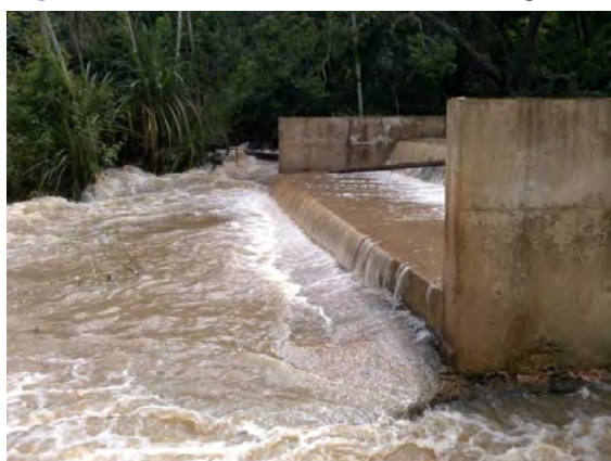
Figure 7. More details on the existing weir
