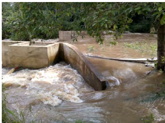
Figure 6. Existing infrastructure situated 1.5km upstream the proposed weir location. Water was overflowing both sides of the weir (March 2017)
