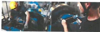
A technician assesses the condition of the gearbox via video endoscopy.
