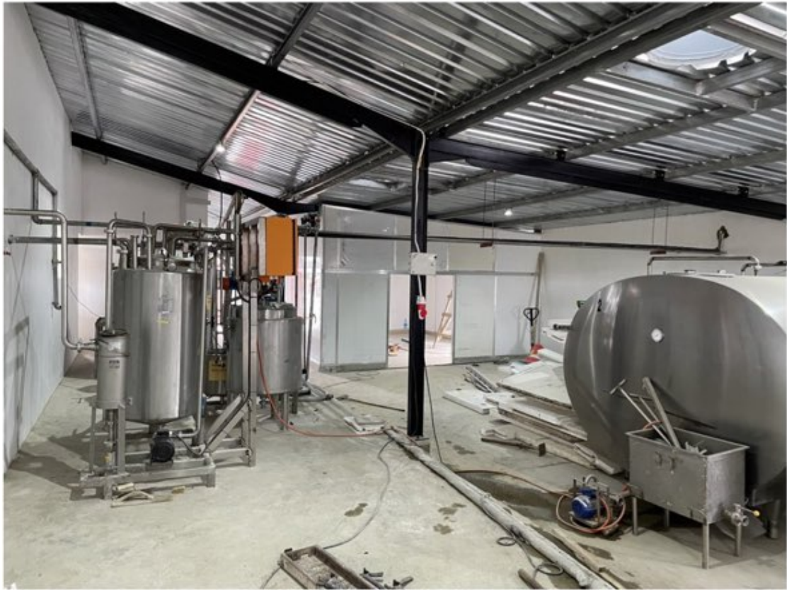
Milk Processing Facility under construction
