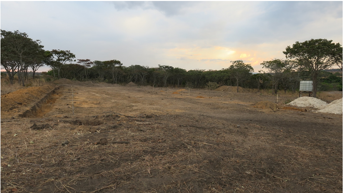
New Dairy Site – Construction in Process
