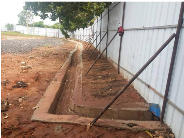
Drainage ditch @ Factory
