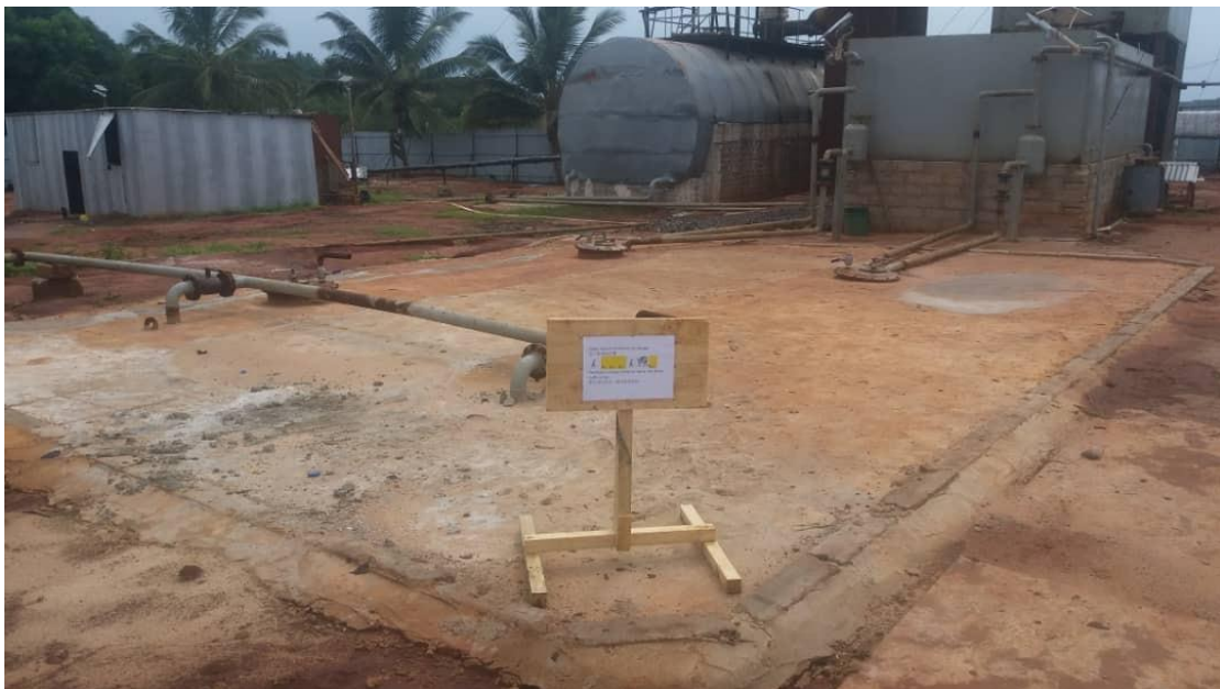
Sign Board @ Ground Top of Under Ground Preliminary Oil Storage Tanks.
