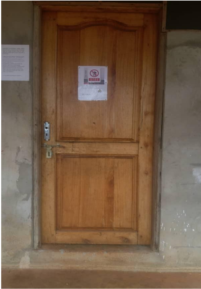
Cautions @ Control Room.
