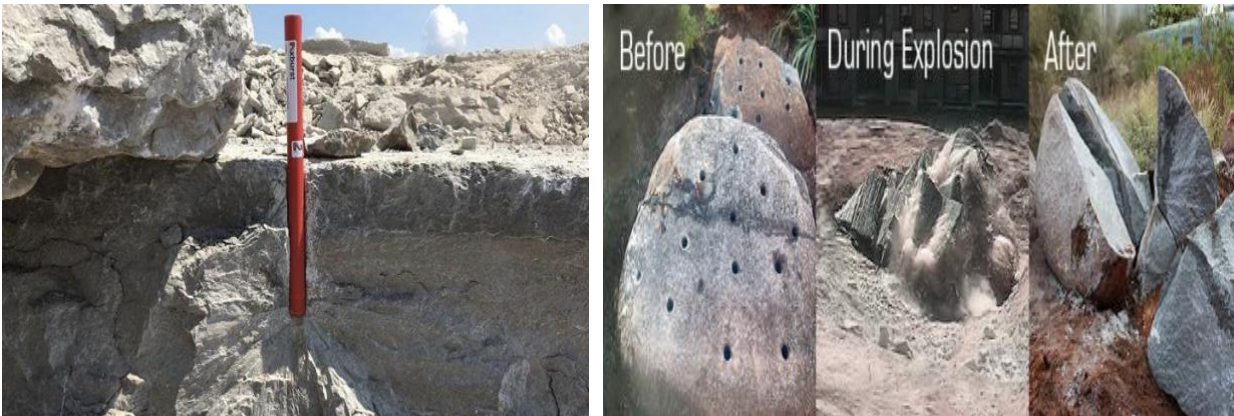
Rock Blasting process
