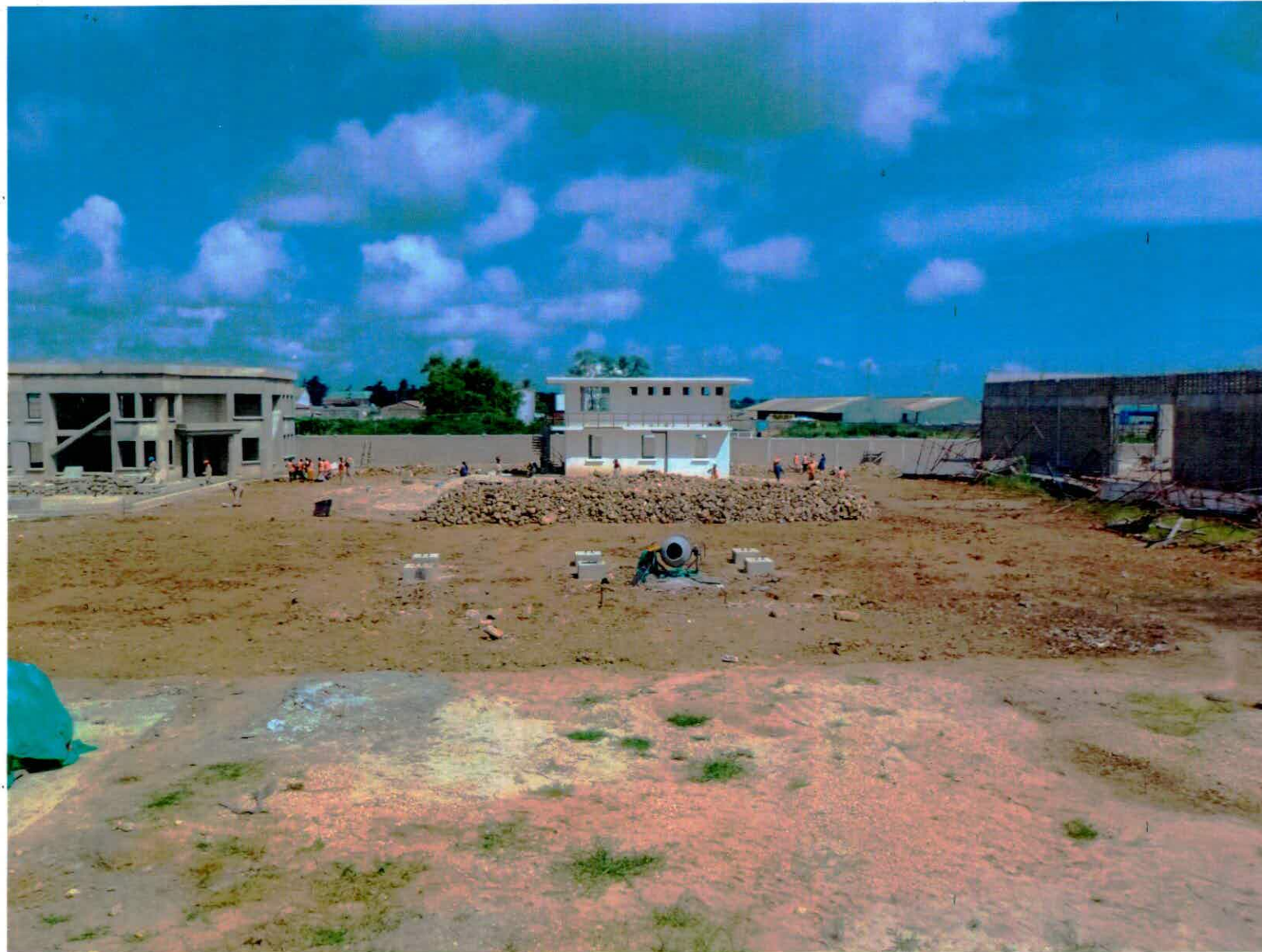
General veiw of admin. Custom offices wearhouse buildings.
