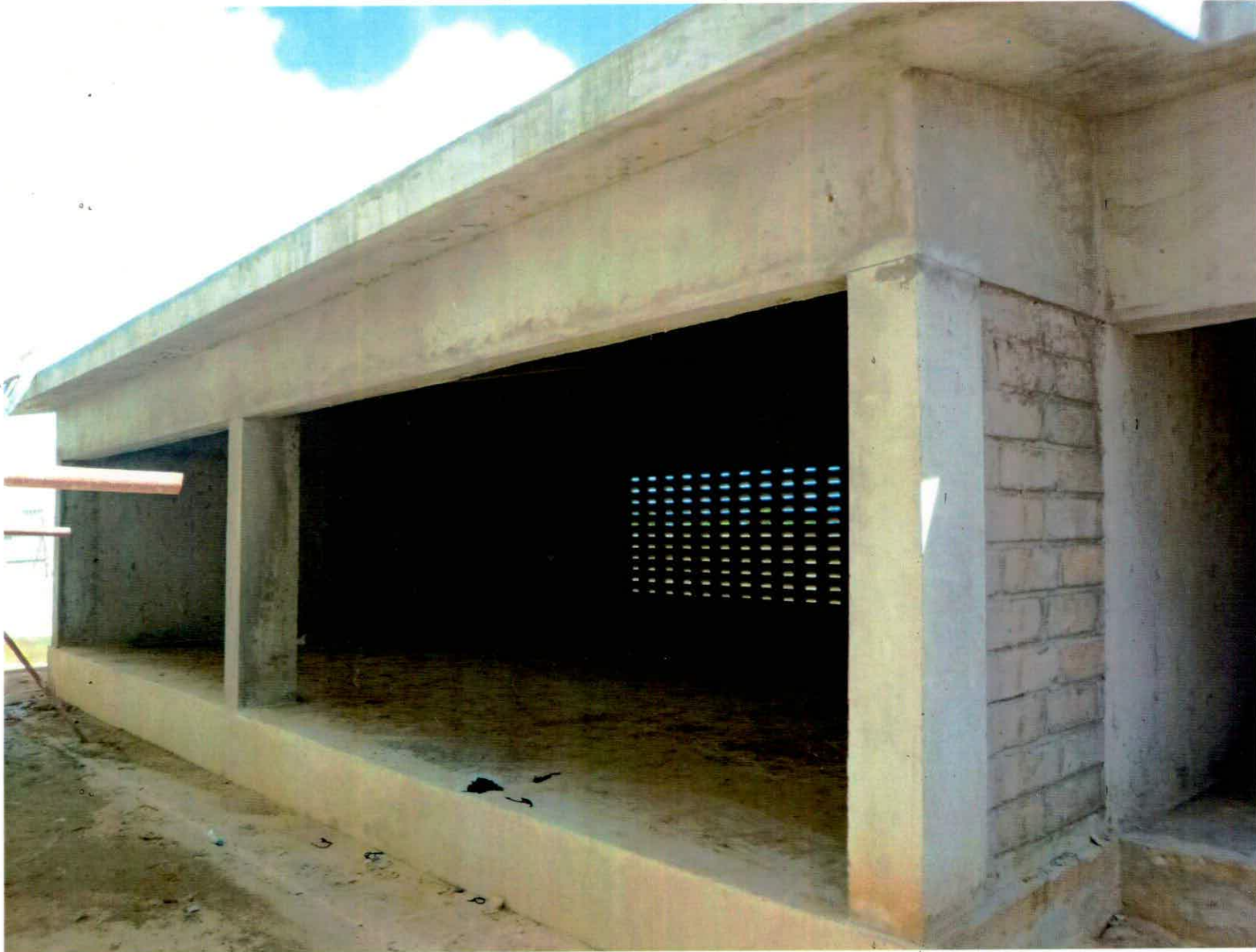
FF pump room
