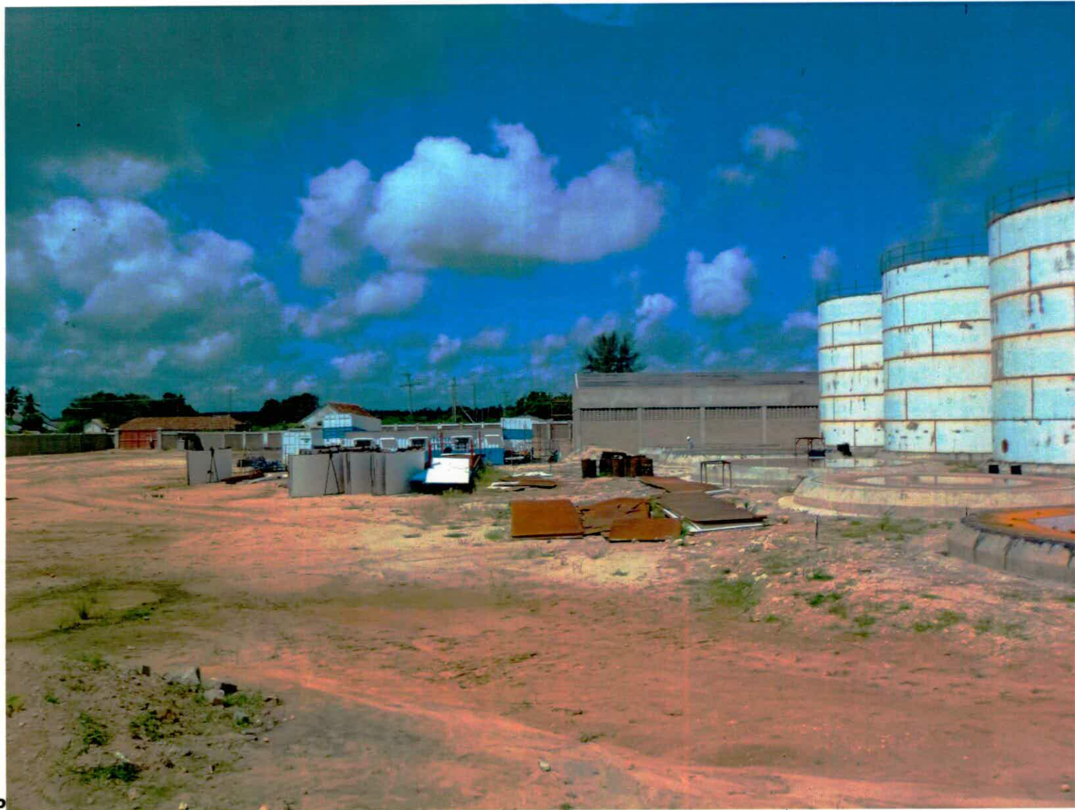
Tank plates + civicon co. offices, phase II area
