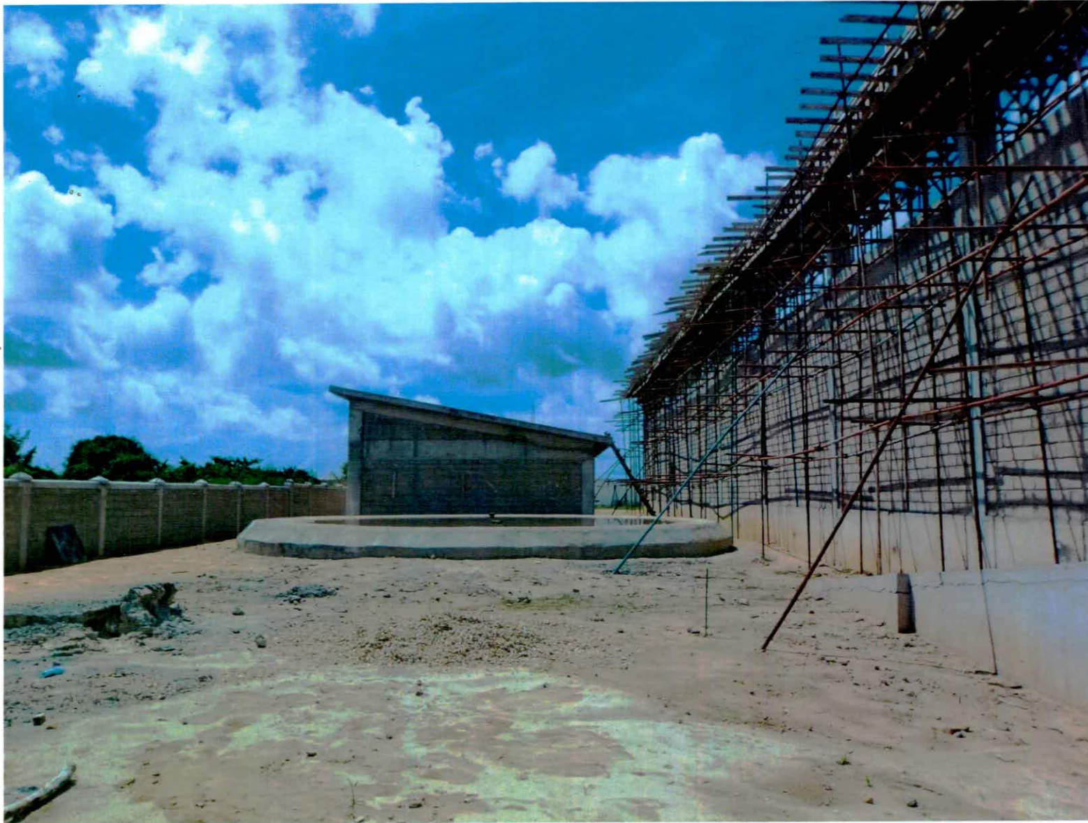
Fire Fighting tank foundation
