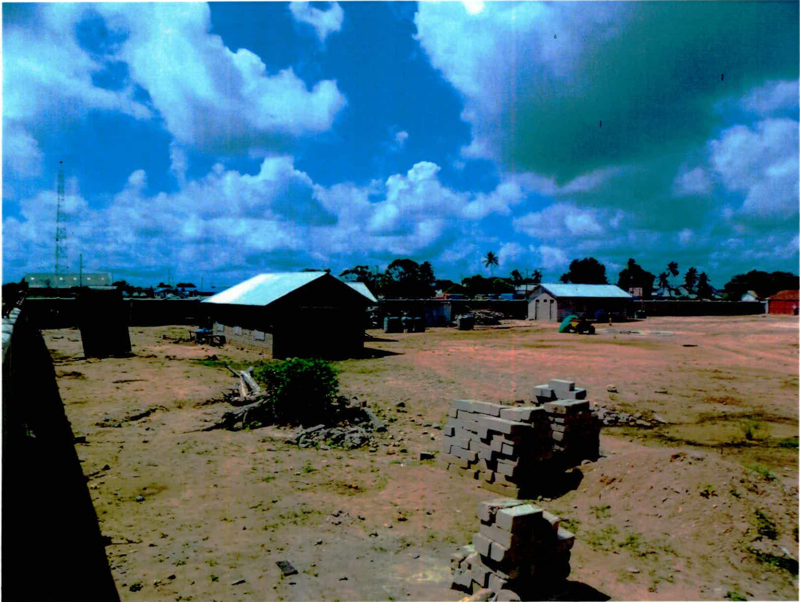
Phase II area / Shibata co. camp.
