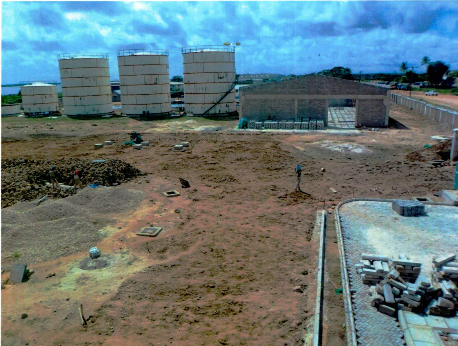
Drum storage /Empty drum shed.
