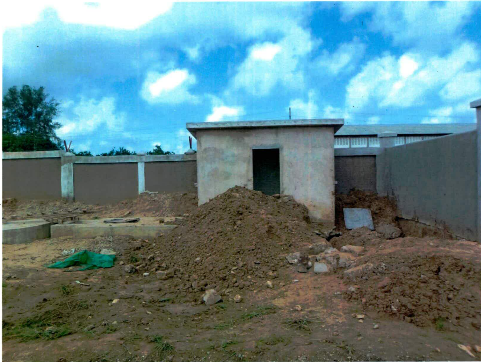
New electric room + generator location, septic tank.
