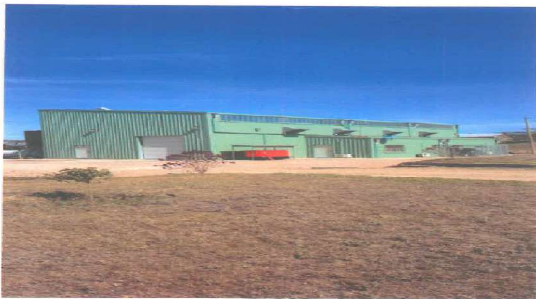
Diesel Power Generators in Loliondo, operated by Tanesco
