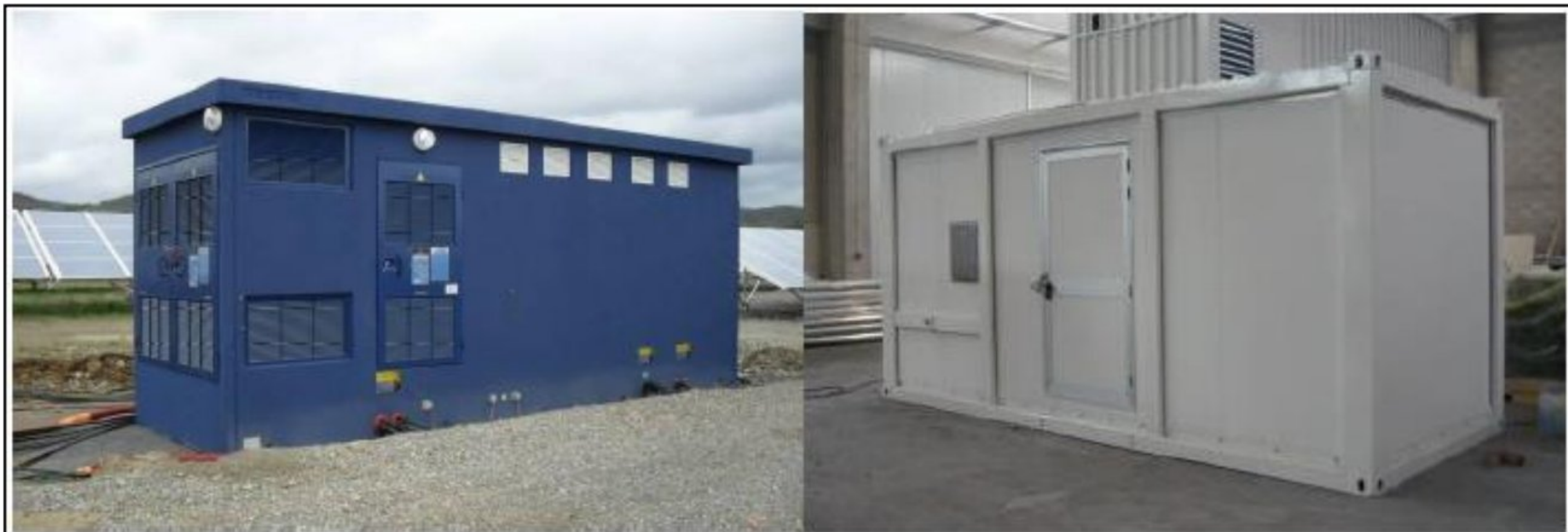
Examples of concrete and container distribution substations
