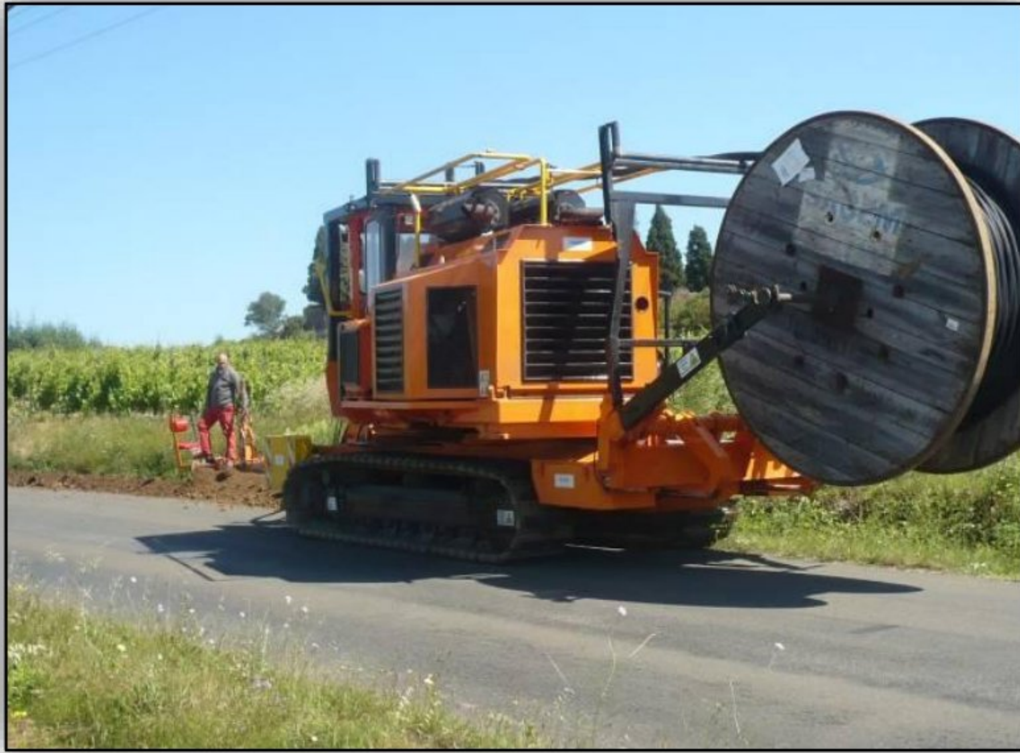
Burying the cable using a trencher
