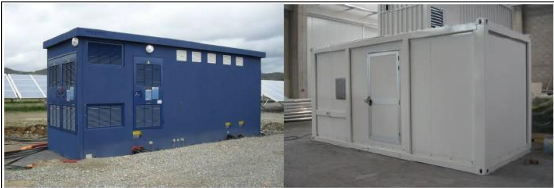
Examples of concrete and container distribution substations
