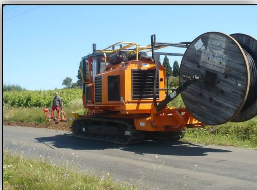
Burying the cable using a trencher
