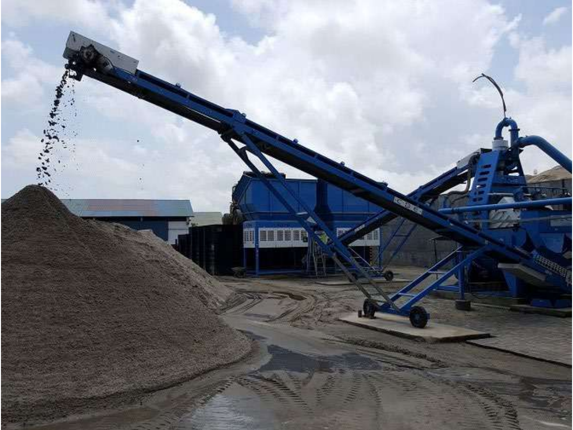
Figure 2: Example of a modern sand washing plant in operation
