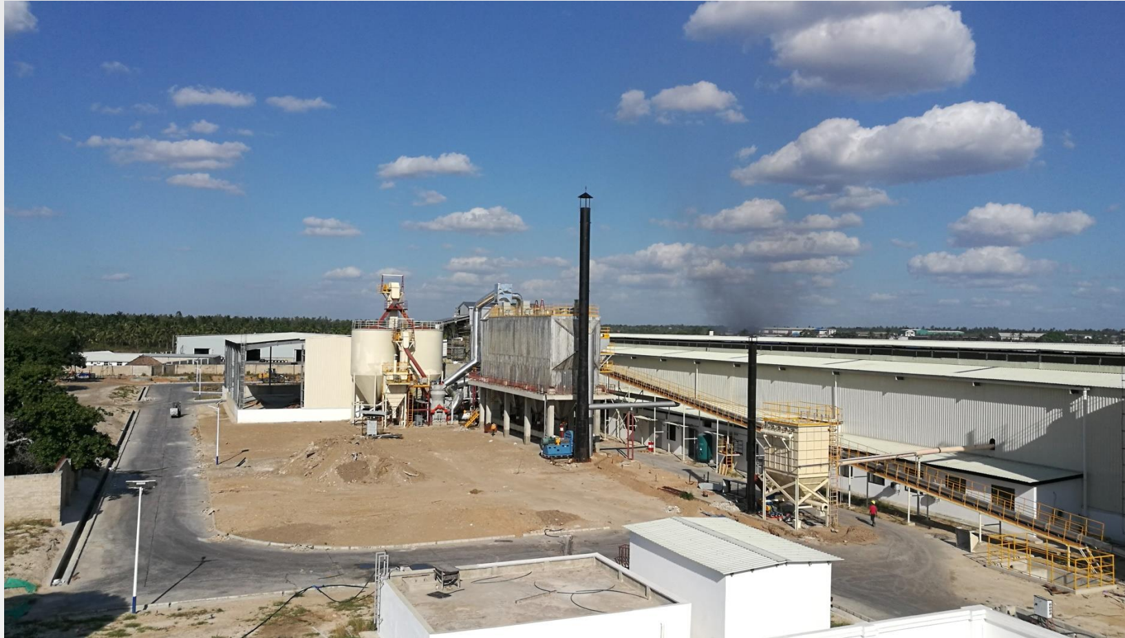
Gypsum Crushing Machine
