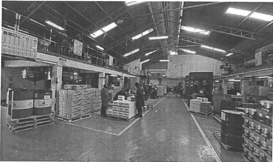
A) Solvent Based Paint Production
