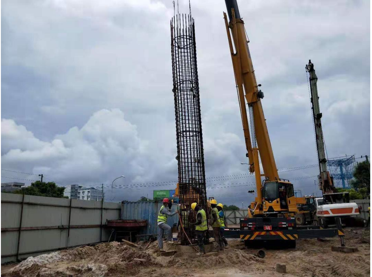
Tanpile at Construction site.
