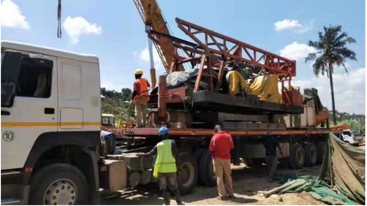
Tanpile at site.
