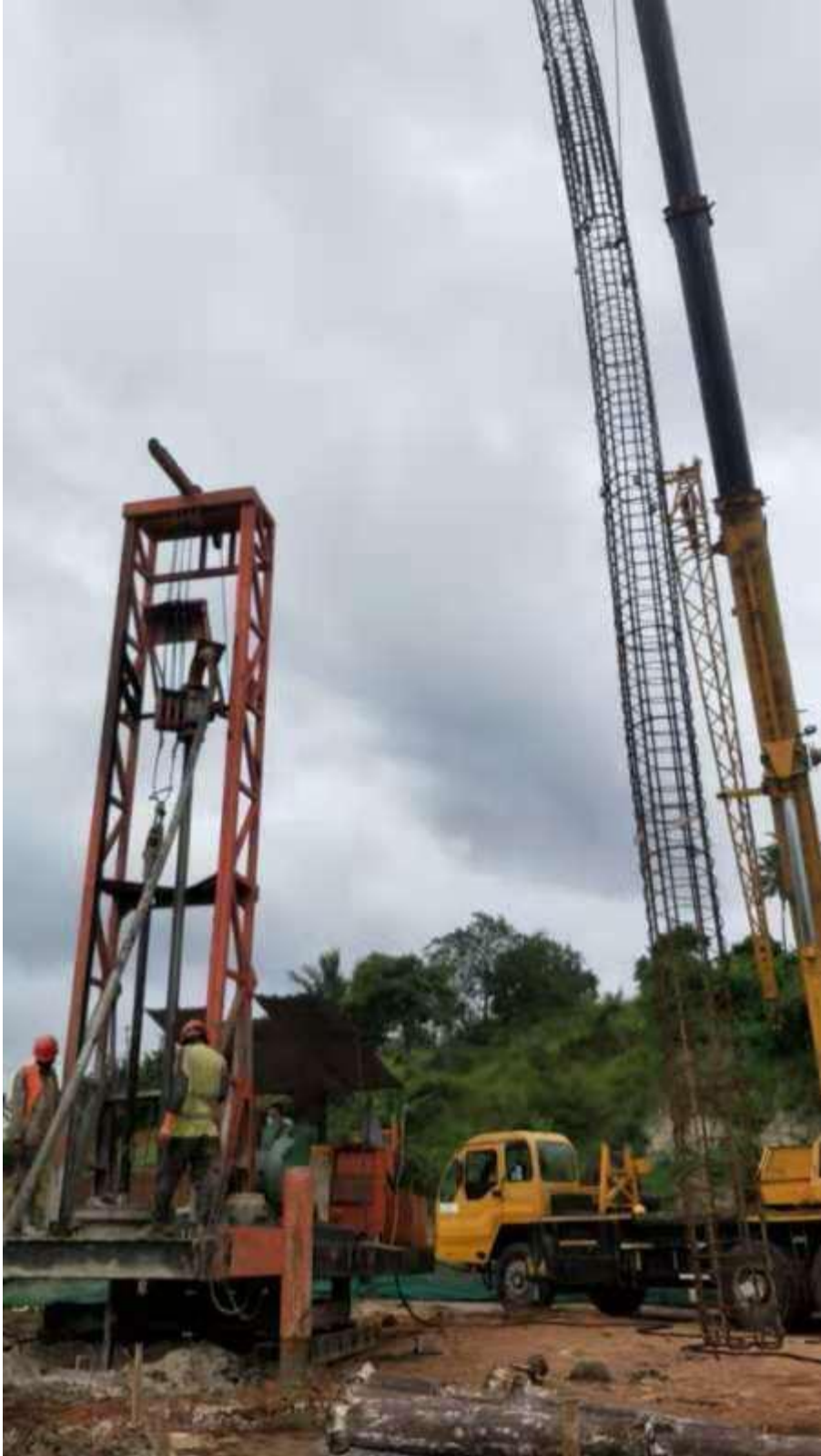
Tanpile at construction site.
