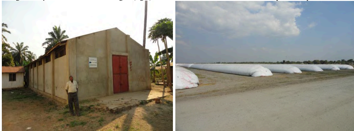
Figure 0.3: A renovated smallholder warehouse at Ifakara, with TAP Extension Officer Elia Shemto (left) and large-scale storage under plastic tunnels at KPL Mngeta (right). The smallholder renovation was funded by the European Union
