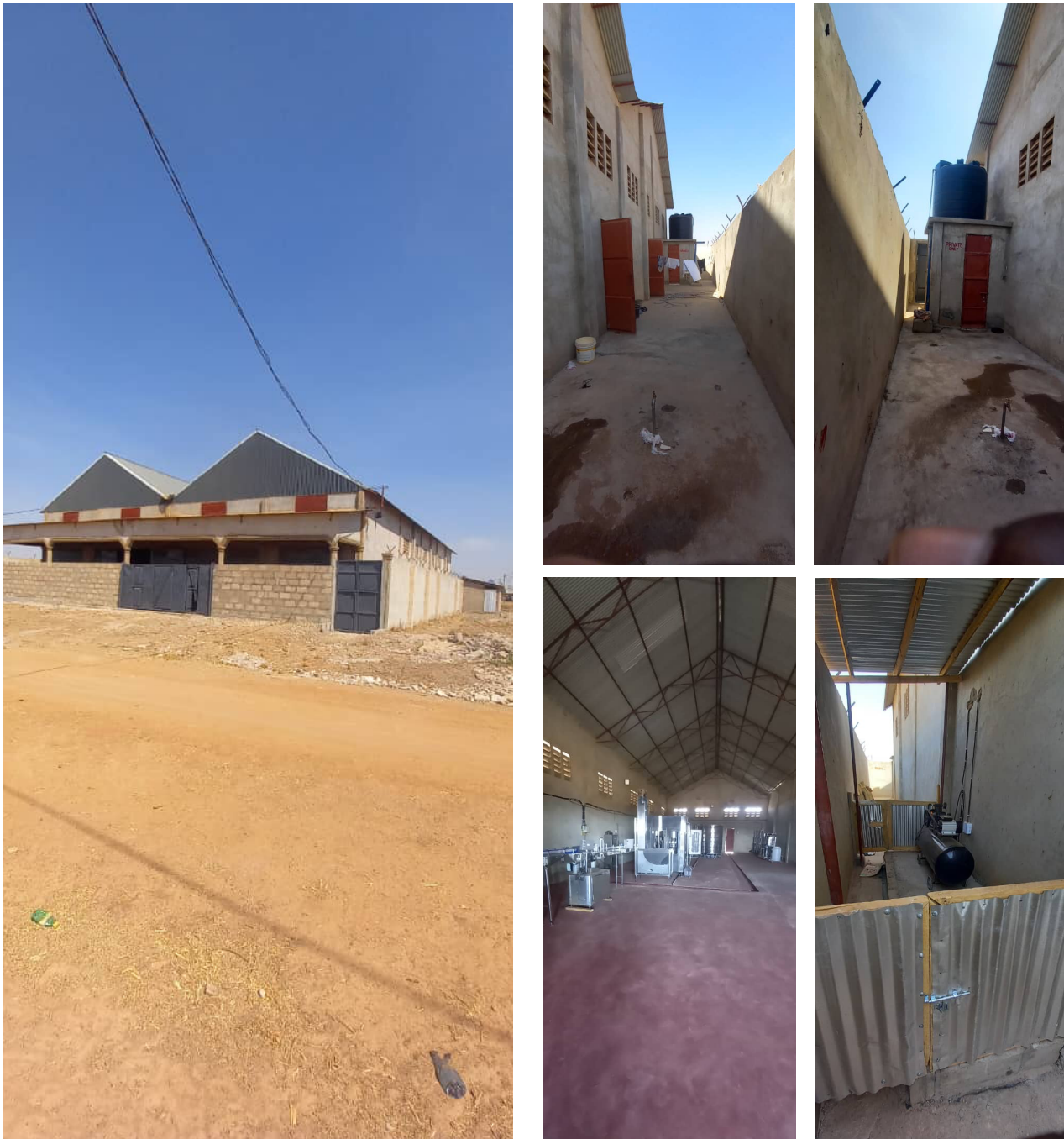
Figure 1 . factory premises outside view and then figure 2 & 3 factory premises backyard, Figure 4 , factory inside one warehouse and then figure 5 is outside factory that houses the Air compressor.
