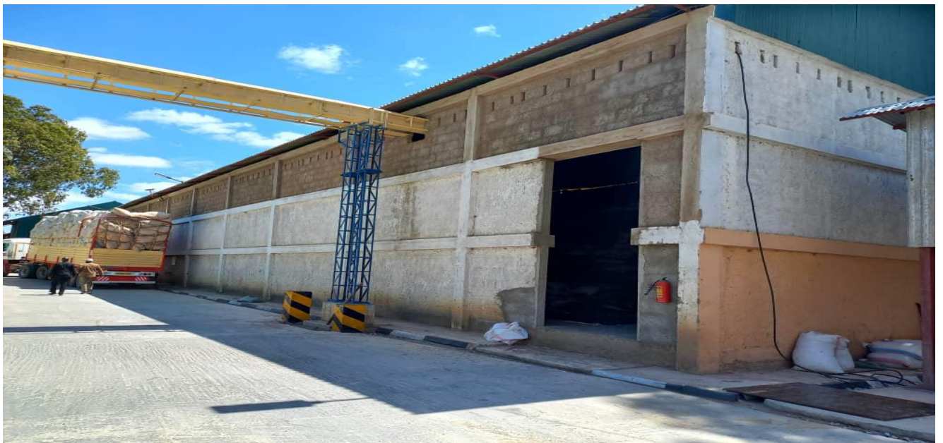
Godown for machinery installation
