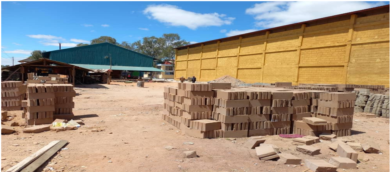
On-going construction of building for installation of double refinery machinery
