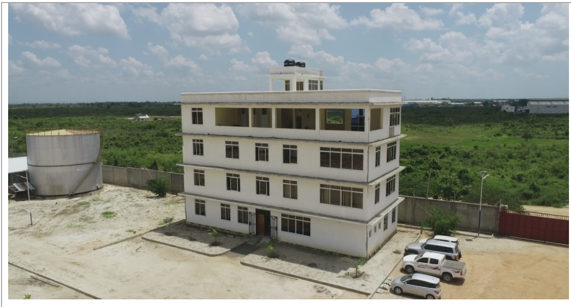
Figure 2: KPIL Superstructure construction progress in pictures
