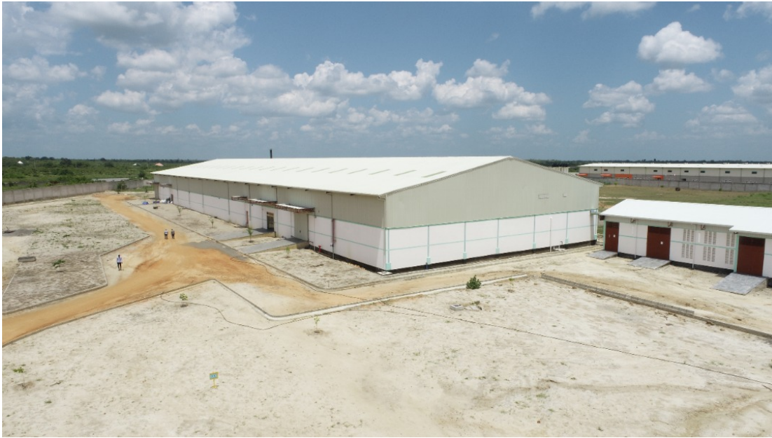
Oblique View of the Factory Building and Powerhouse; April 2022
