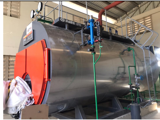
Figure 2 installation of 8tons boiler
