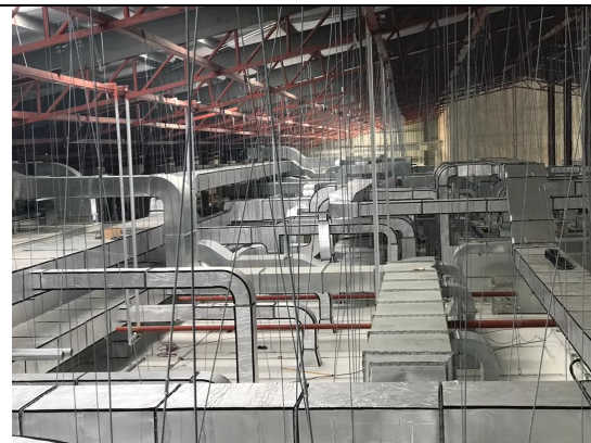
Figure 4 AHU ducts works on progress
