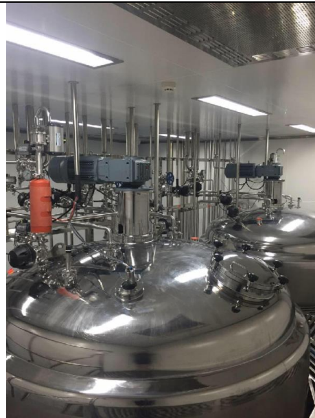
Figure 3 Solution preparation tank at site
