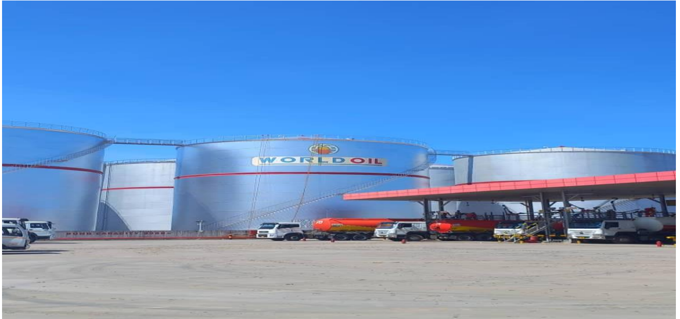
Petroleum storage Facilities and filling station
