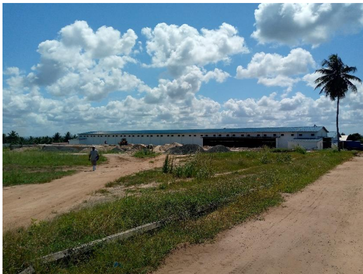
Construction of additional poultry units, Layers Farm
