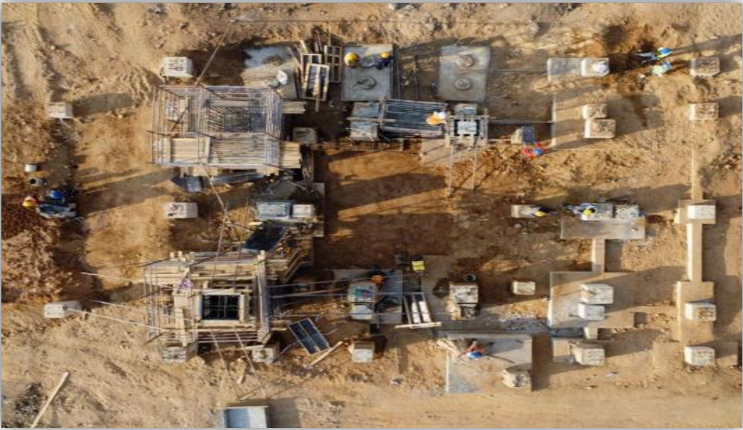
Boiler piles, foundations and plinths /
