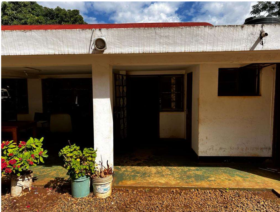
Main entrance to the Office Building
