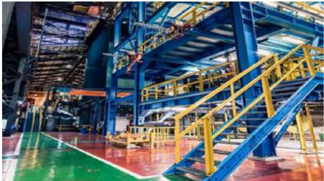
Aluzinc coating plant
