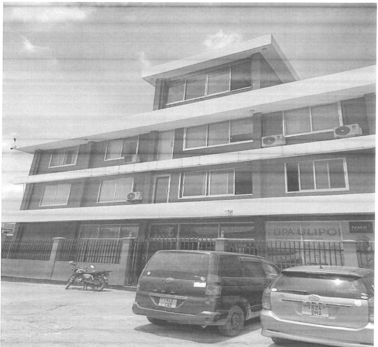
Office building for the project
