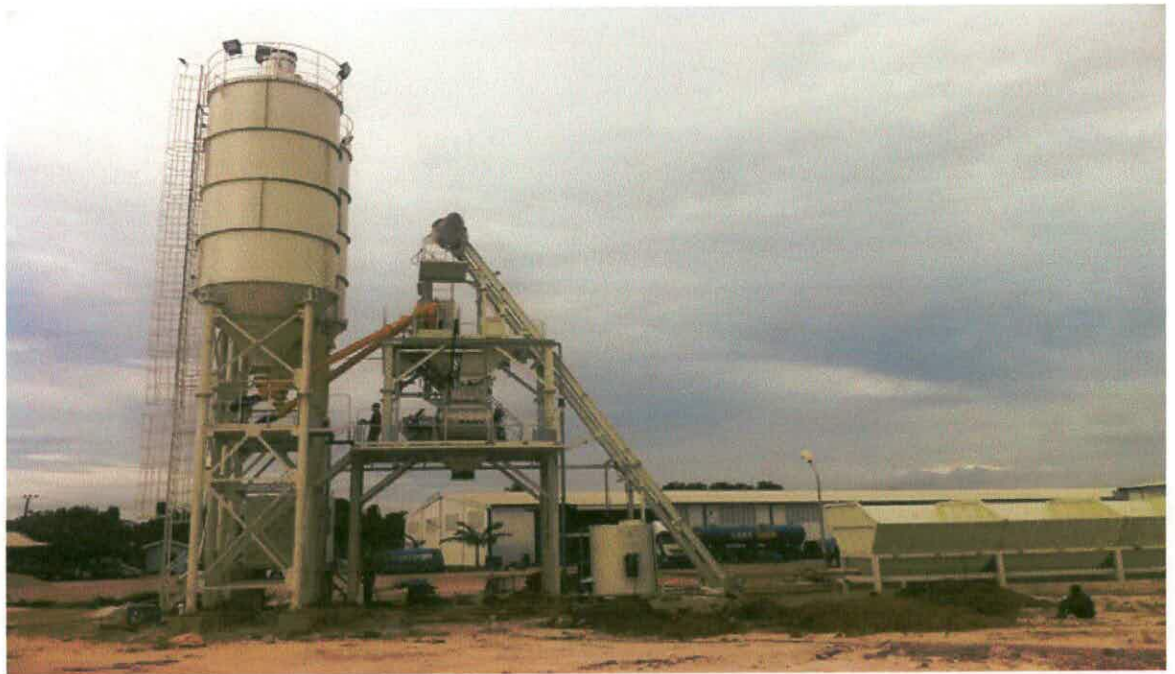
Cement Silo in Mikocheni Plant
