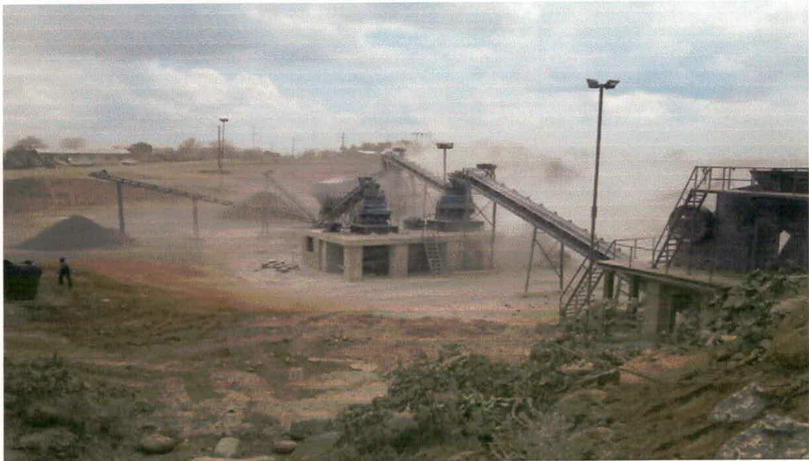
Crusher in Lugoba Quarry
