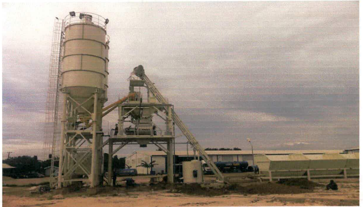
Cement Silo in Mikocheni Plant
