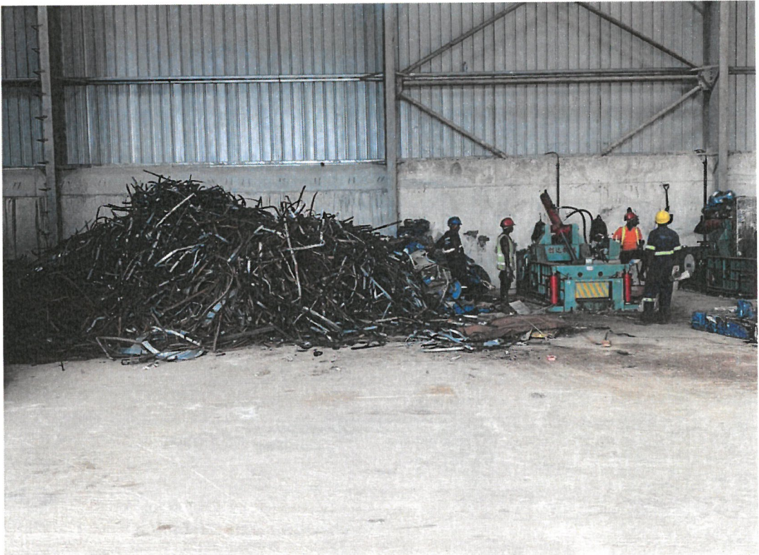
New Shades for storage of scrappers which is under constructions
