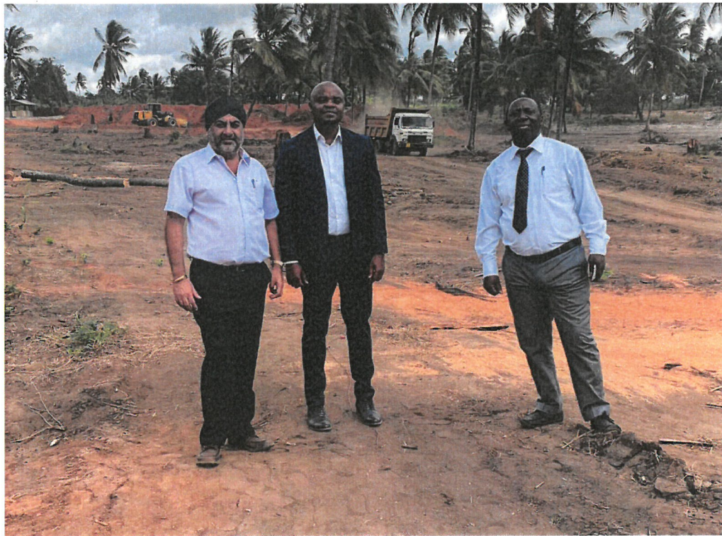
Lodhia Steel Industries Ltd General Manager from left Mr. ...., Aftercare Manager tClearance of the new area for extension of the Manufacturing plant
